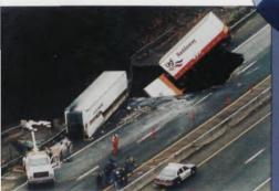
Days of abnormally heavy rains in November undermine the roadbed of Oregon's Interstate 5, creating a 40-foot-deep sinkhole, into which two semitrailer trucks tumble.
